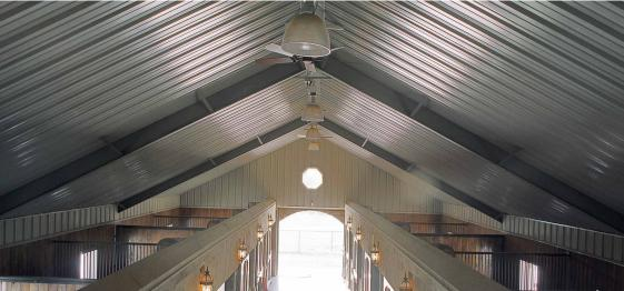
The PBR panel is commonly used for a wide variety of architectural, agricultural, commercial and industrial applications. PBR is a structural panel and an exposed fastener panel that can be used for both roof and wall applications. The minimum roof slope for PBR is ½:12.
