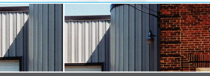
The AVP panel is used for wall application and features pencil ribs, providing improved aesthetics to the building design.
