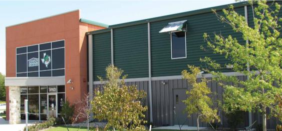
The PBU panel is an exposed fastener system for wall applications. PBU can be installed directly over purlins or joists. PBU offers the versatility of being used in both vertical and horizontal applications to give designers a contemporary appearance for their building project. PBU is recommended for 1:12 or greater roof slopes.
