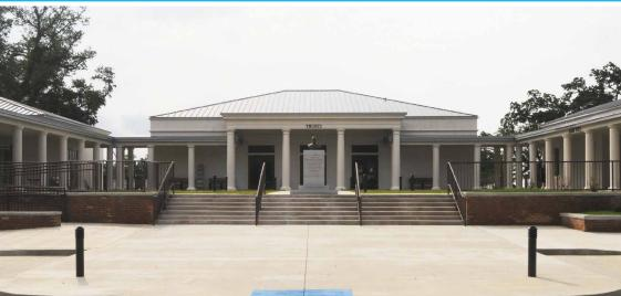
BattenLok® HS is a mechanically field seamed, high strength structural standing seam roof system. The BattenLok® HS panels have a 2" tall vertical seam and are available in both 12-inch and 16-inch widths. BattenLok® HS can be installed directly over purlins or bar joists and is capable of transitioning from roof to fascia. BattenLok® HS does not require a solid substructure for support.
