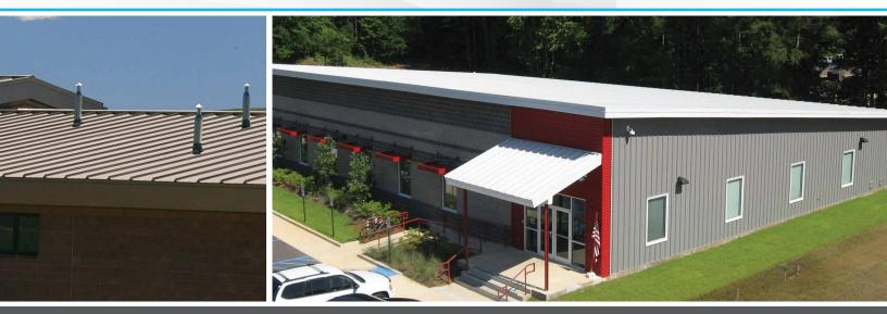
The Double-Lok<sup>®</sup> roof panel is a mechanically field-seamed, trapezoidal leg standing seam roof system. Double-Lok<sup>®</sup> panels are available in 18-inch and 24-inch widths. Double-Lok<sup>®</sup> requires a minimum slope of <sup>1</sup>/<sub>4</sub>:12. Double-Lok<sup>®</sup> panels are ideal for industrial, commercial and architectural applications.
