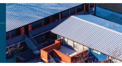
The PBR panel is commonly used for a wide variety of architectural, agricultural, commercial and industrial applications. PBR is a structural panel and an exposed fastener panel that can be used for both roof and wall applications. The minimum roof slope for PBR is ½:12.
