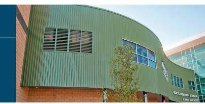
The PBU panel is an exposed fastener system that can be used for both roof and wall applications. PBU can be installed directly over purlins or joists. PBU offers the versatility of being used in both vertical and horizontal applications to give designers a contemporary appearance for their building project. PBU is recommended for 1:12 or greater roof slopes.
