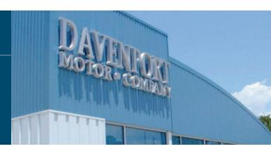
ShadowRib<sup>TM</sup> is a 3" deep panel that combines aesthetics, economy and function to bring definition to metal structures. ShadowRib<sup>TM</sup> is a proven performer and a versatile tool to the designer. Structural strength in the ShadowRib<sup>TM</sup> panel is accomplished without sacrificing appearance or design flexibility. The fluted face creates distinctive shadow lines.
